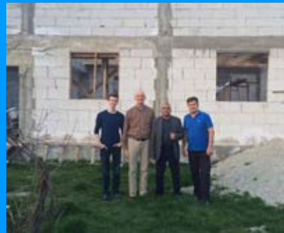
Gypsy Church under construction
